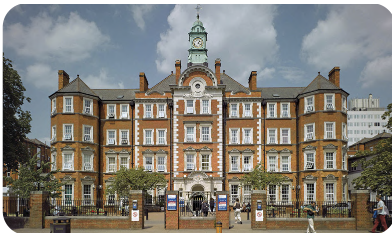
Hammersmith Hospital with the Royal Postgraduate Medical School on the right. © Hammersmith Hospital
